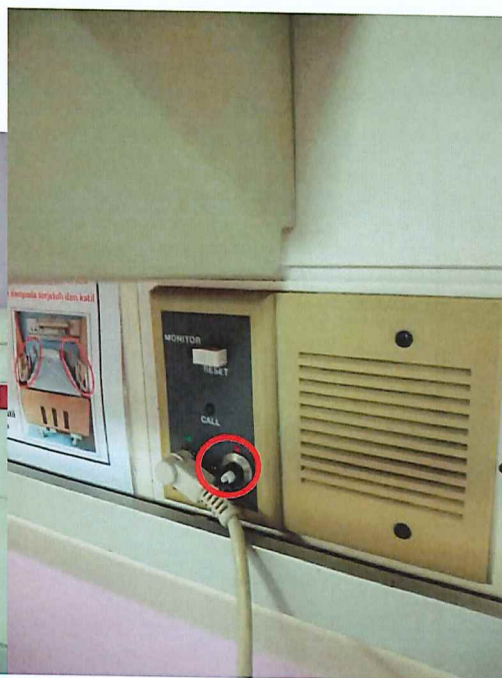
Bed Station for Bed 703A and Bed 704A Found Emergency Button Faulty.
