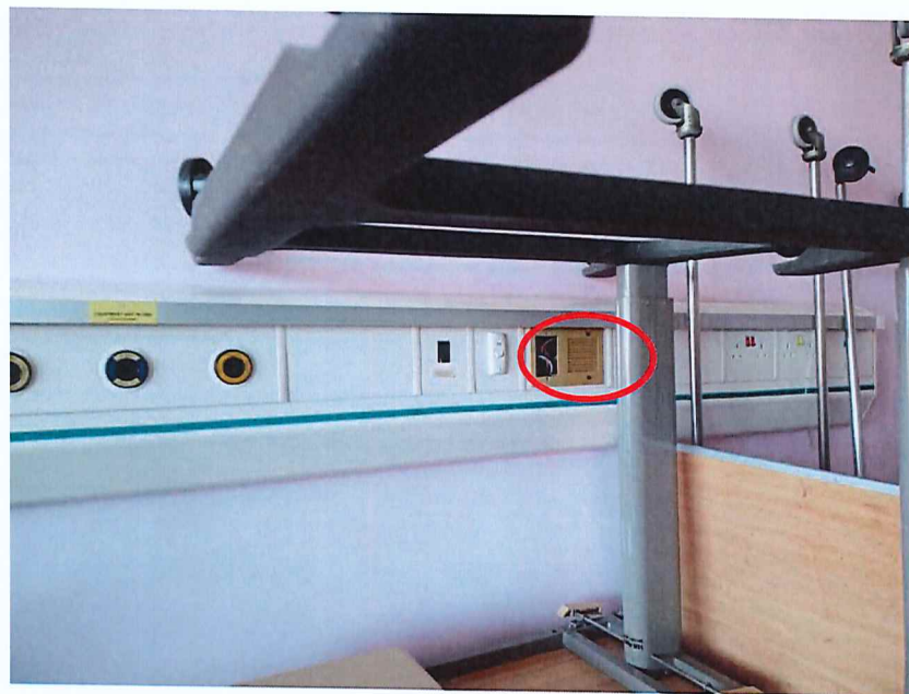
Bed Station and for Room DS1 Found Faulty and Call Cord Not In Place.
