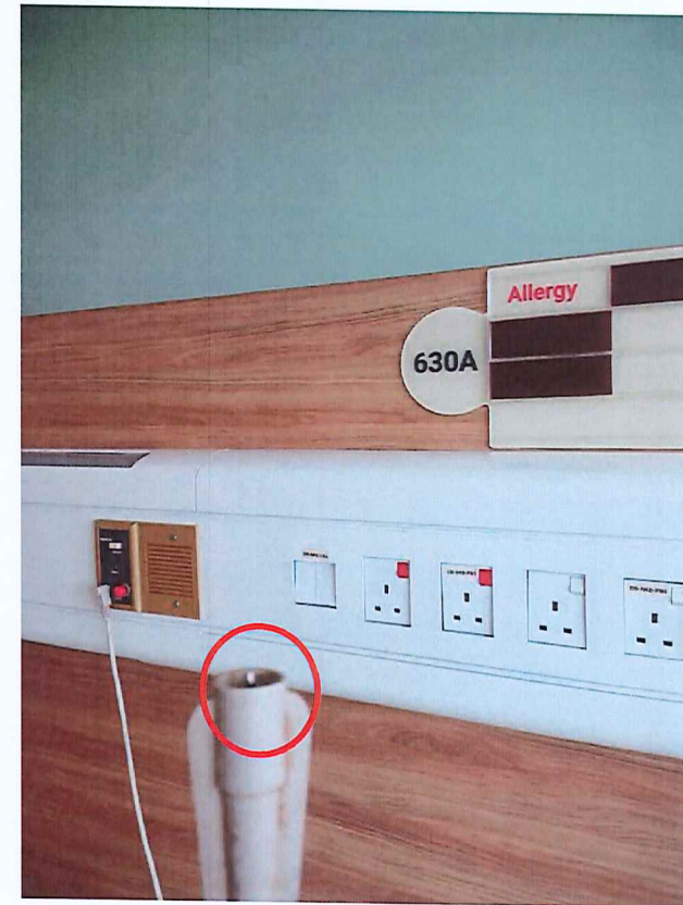
Call Cord Button Not In Place for Room 639D
