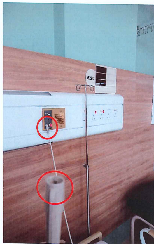
Bed Station for Bed 629C Found Faulty and Call Cord for Button Not In Place.
