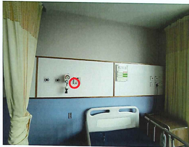
Call Cord Button for Bed 526A, Bed 526B & Bed 526D Found Not In Place.
