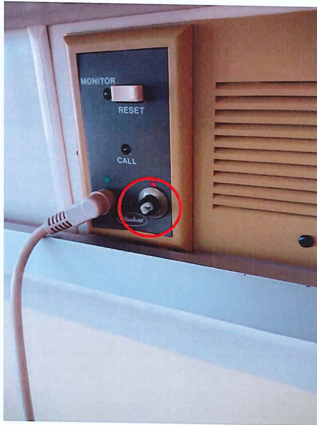
Bed Station for Room 707C Found Emergency Button Broken.
