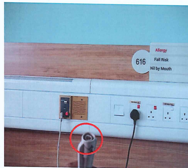
Call Cord for Bed 616 Found Button Not In Place.
