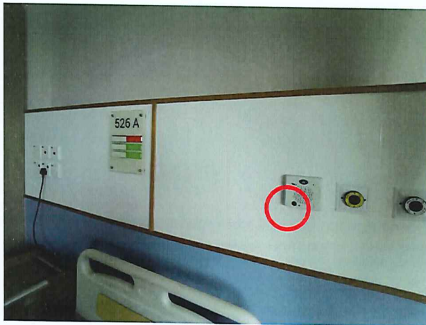
Call Cord Button for Bed 526A, Bed 526B & Bed 526D Found Not In Place.
