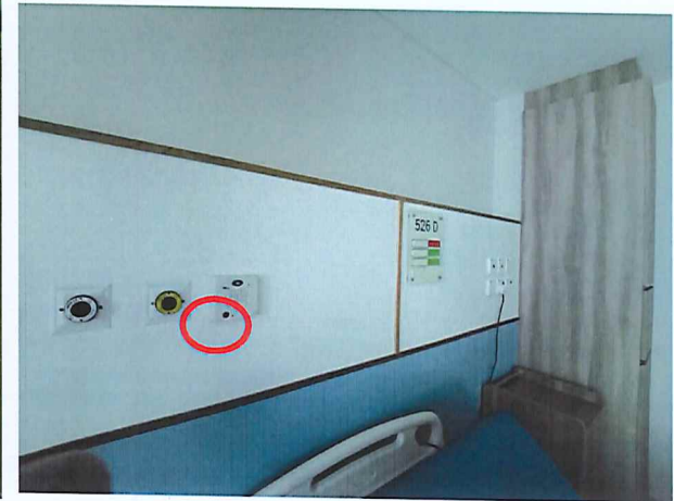
Call Cord Button for Bed 526A, Bed 526B & Bed 526D Found Not In Place.
