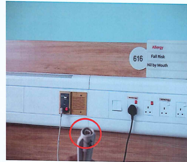
Call Cord for Bed 616 Found Button Not In Place.
