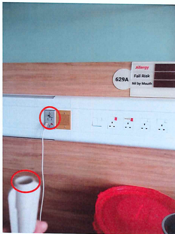
Bed Station for Bed 629A Found Faulty and Call Cord for Button Not In Place.
