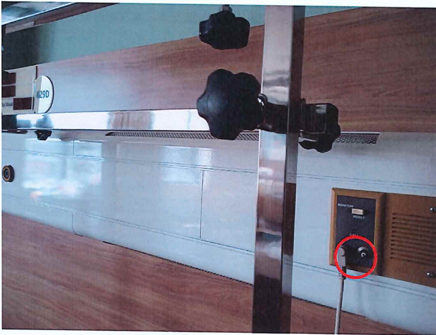
Bed Station for Bed 629D Found Emergency Button Faulty.
