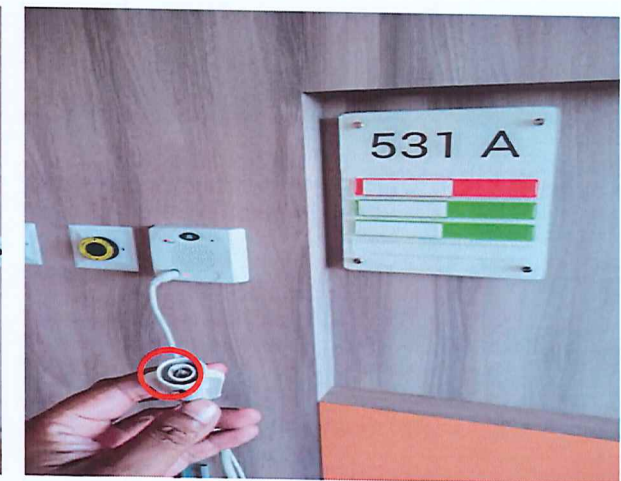
Call Cord Button for Bed 531A Button Not In Place.
