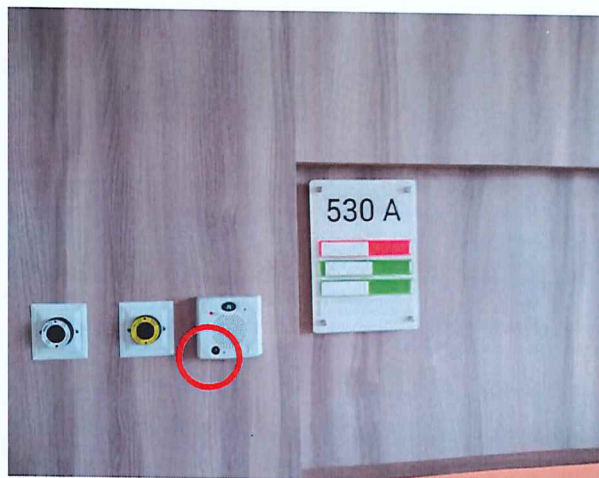
Call Cord Button for Bed 530A & Bed 530B Found Not In Place.
