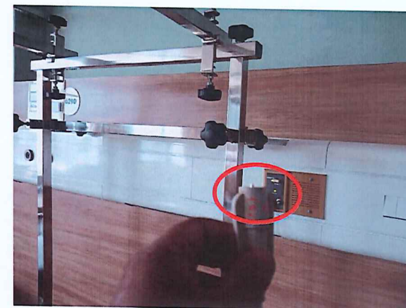
Call Cord Button Not In Place for Room 630A
