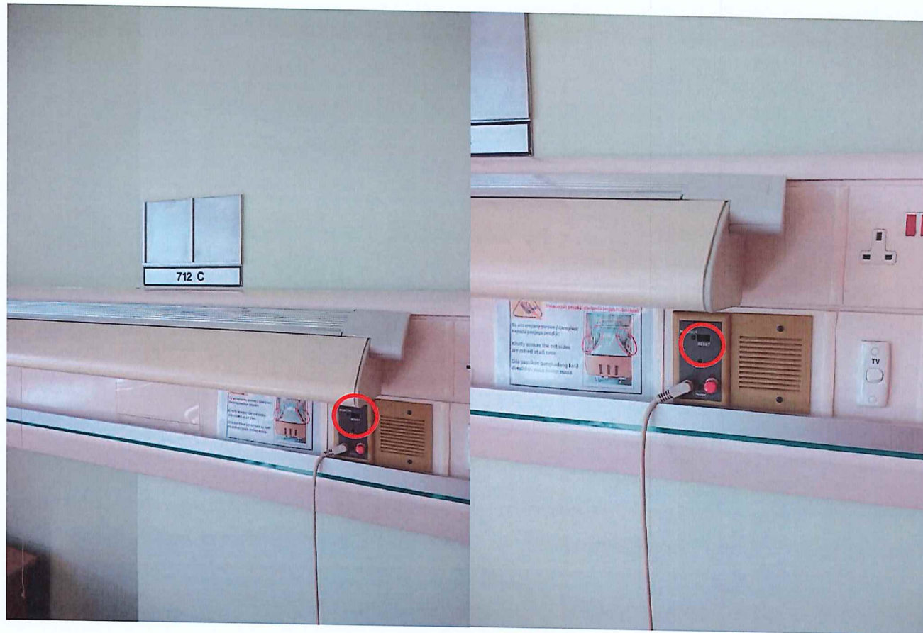
Bed Station for Bed 712C Found Reset Button Not In Place.
